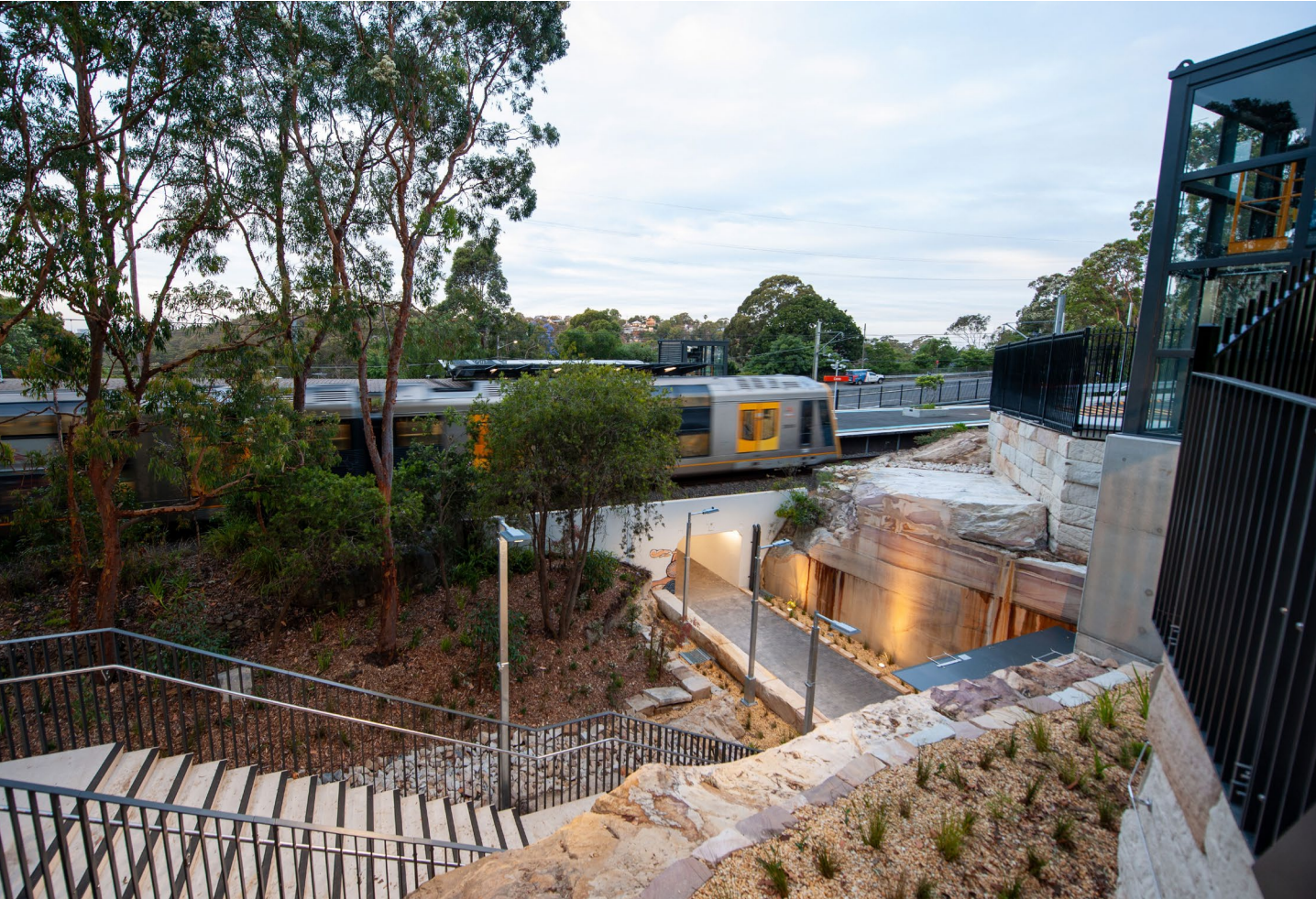
Como Station upgrade ©Transport for NSW
